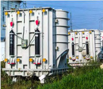
60MVar/500kV Shunt Reactor Tulum Substation, Russia
