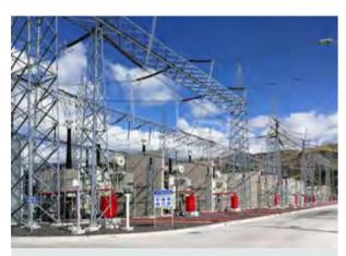
250MVA-500kV Transformer Inga Substation Ecuador
