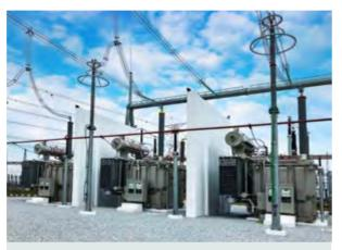
350MVA-500kV transformer Olak substation Malaysia
