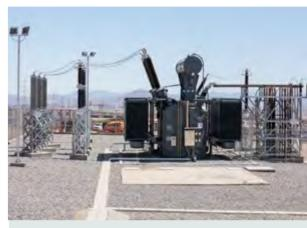
230MVA-220kV Transformer El Romero Substation Chile
