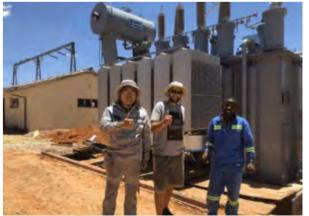
50MVA-132kV Transformer Nyanga Substation Zimbabwe
