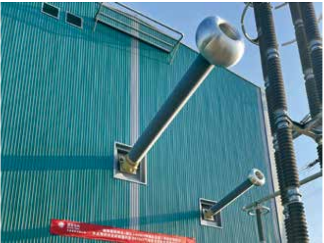
• ±800 and ±400kV DC wall-through bushing, Wuhan, China
