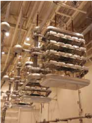
• ±800kV DC converter valve lightning arrester
