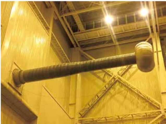
• ±1100kV DC wall-through bushing, Changji, China
