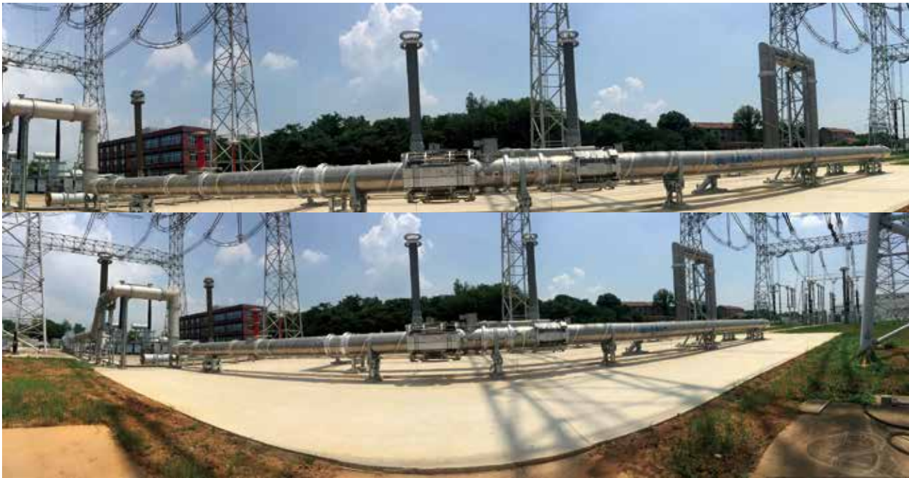
• Eco-friendly 1000kV GIL State Grid Ultra High Voltage AC Test Base
