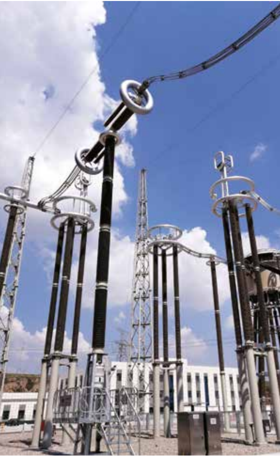
• 816kV DC bypass switch (Shaanbei converter station)
