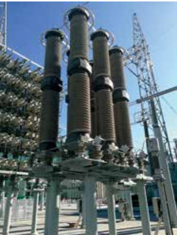
• +11000kV CNB2 lightning arrester
