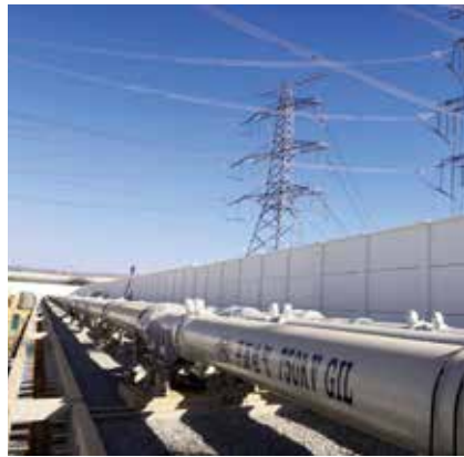
• 800kV GIL China Shanxi Baoji substation
