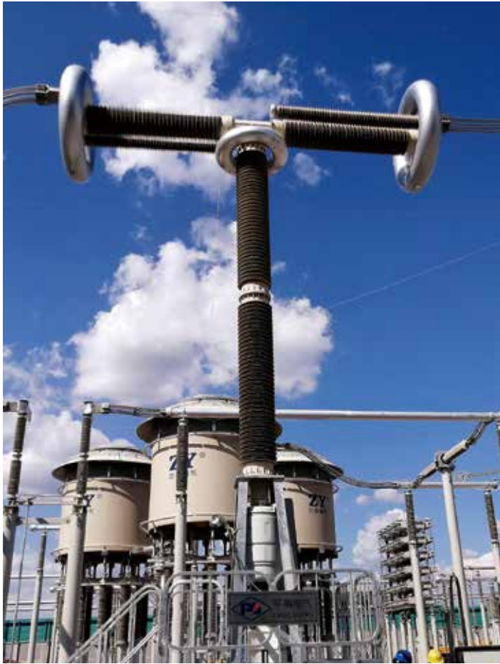
• 408kV DC bypass switch (Shaanbei converter station)
