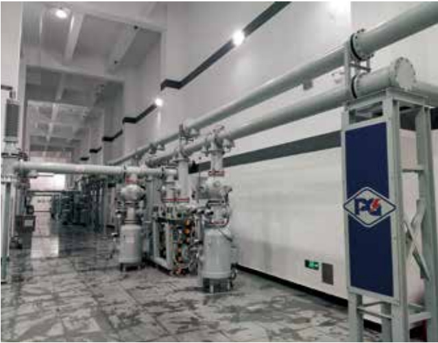
• 72.5kV low frequency GIS,Zhejiang,China
