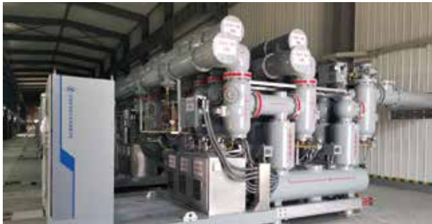
• Qingcheng 252kV 63kA GIS, Guangdong, China
