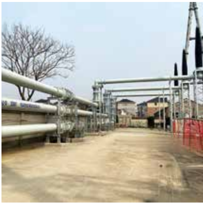
• 550kV GIL China Zhejiang Chaoyong substation
