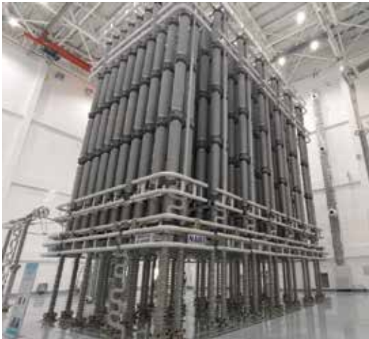
• ±800kV self-healing energy dissipation arrester
