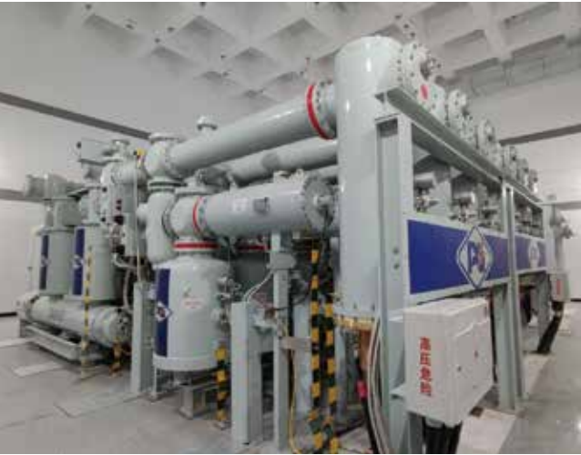
• 252kV low frequency GIS, Zhejiang,China
