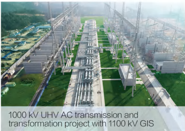
1000 kV substation expansion project with 1100 kV GIS
