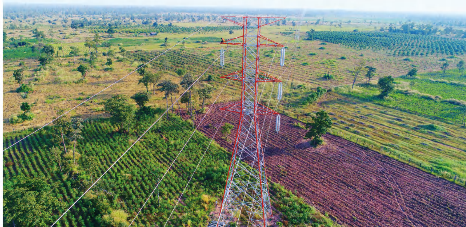
©PEA' s first public works demonstration project for distribution network upgrade
