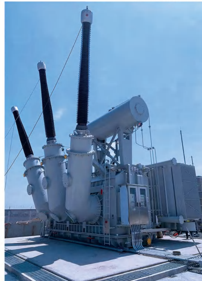
400kV, 165MVA three-phase transformer at the Santa Cruz New Energy Substation in Mexico
